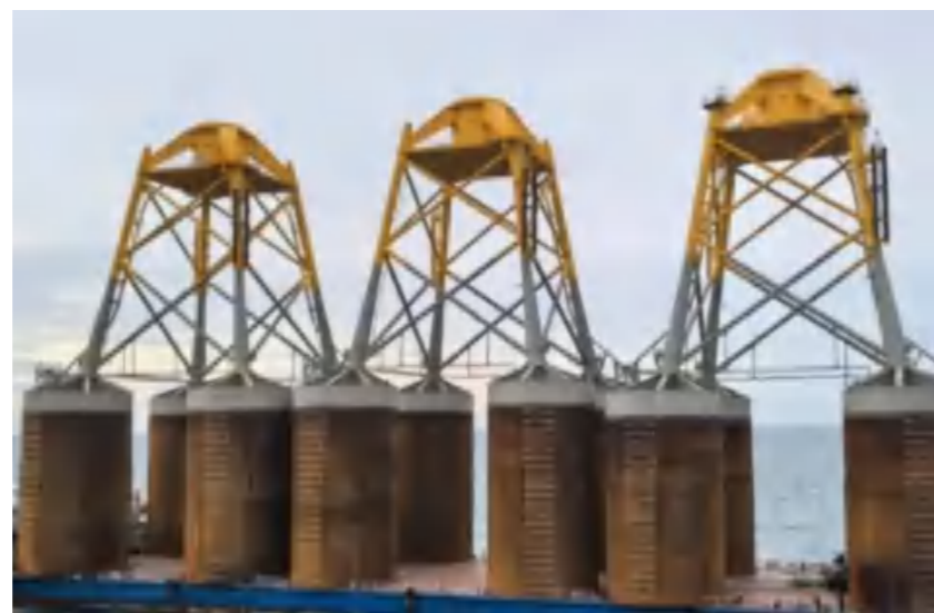
Sucking Bucket Offshore Wind Jacket China Datang CZ3 Offshore Wind Farm Project, Danzhou City, Hainan Jacket and Monopile 10MW
