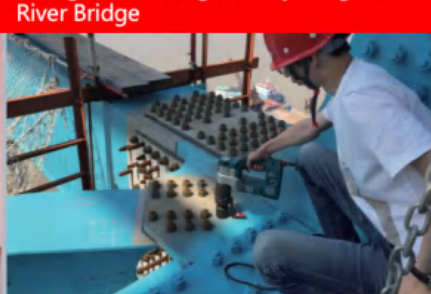
Shanghai-Nantong Railway Yangtze River Bridge
