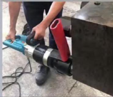
TCD10000 installation of breaker hammer
