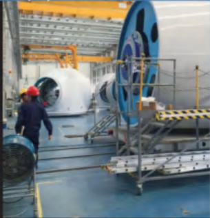
Wind power equipment installation
