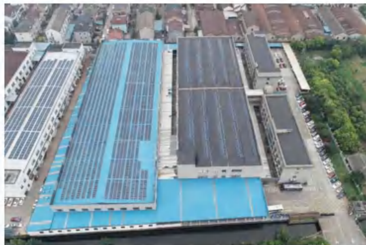
宁波工商业电站7.5MWP
