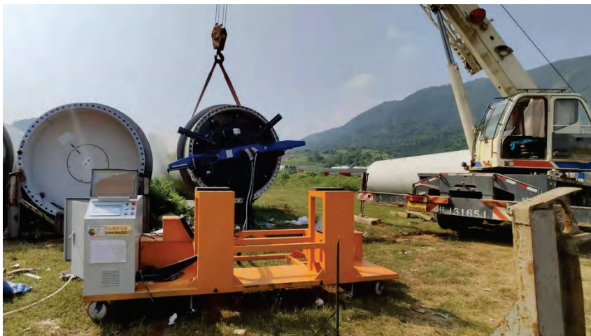
Fig. 12 Rework the blades in the wind farm
