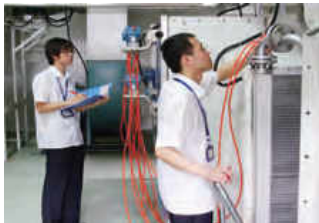
Performance Test 换热性能试验
