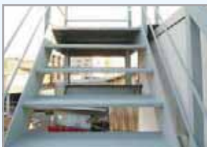
Exterior steel stairs
