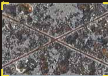
Rust from cross-cut spreads.
