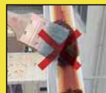
Applying product to rusted surfaces
