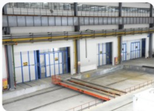
Tank Coating Line
